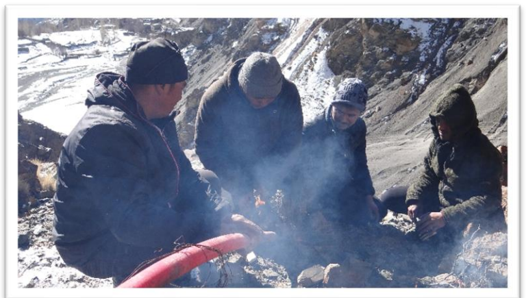
Zomal villagers installing pipes for their Artificial Glacier
